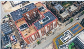
Nordhavn rooftop solar panels
